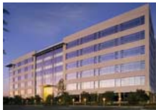
Timberline Commercial Real Estate in partnership with SE Corp. has developed a 160,000-square-foot office tower in Lakeshore Plaza in the Dos Lagos community of Corona, Calif.
