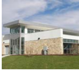
KAI Design & Build is nearing completion of its $10.5 million Southeast Community Center project located in Kansas City, Mo.
